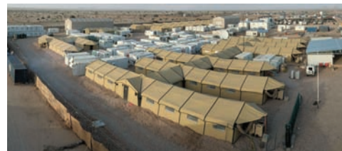
Fully laid out Norwegian deployable Hospital, the white containers in the centre is the Marshall supplied Role 2 hospital.
